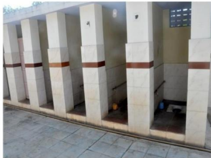
Boys Toilet - Western side
