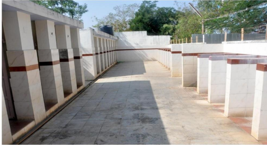
Girls Toilet - Eastern side
